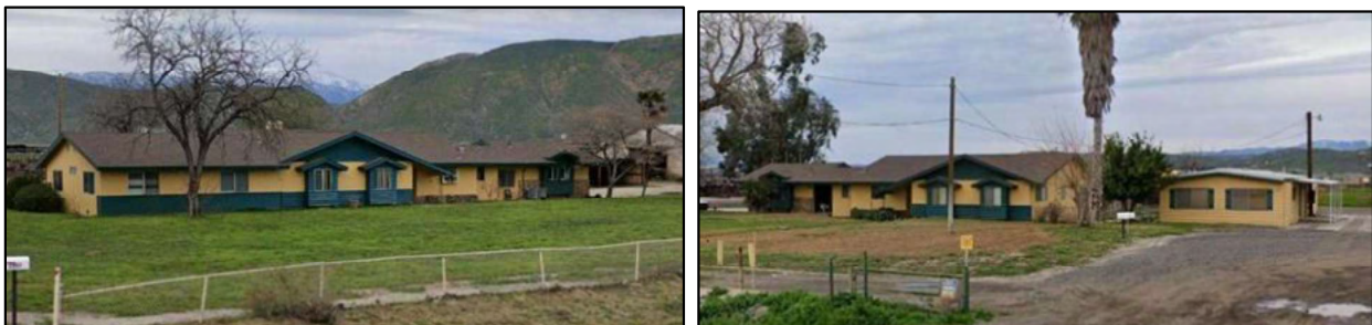
Figure 36. Ramona Dairy #1, 2451 Ramona Expressway
