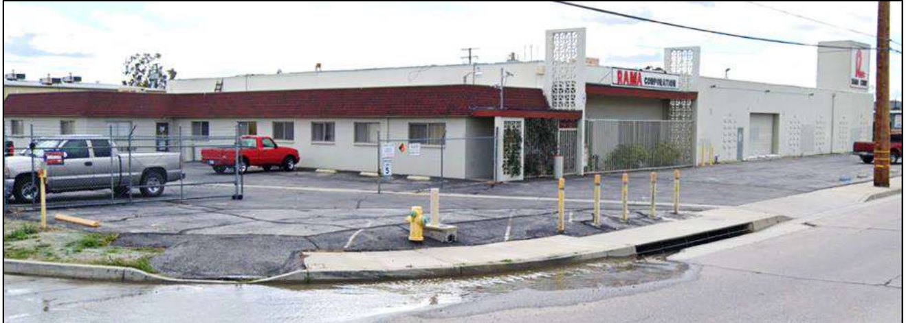
Figure 52. Rama Corp, 600 W. Esplanade Avenue
