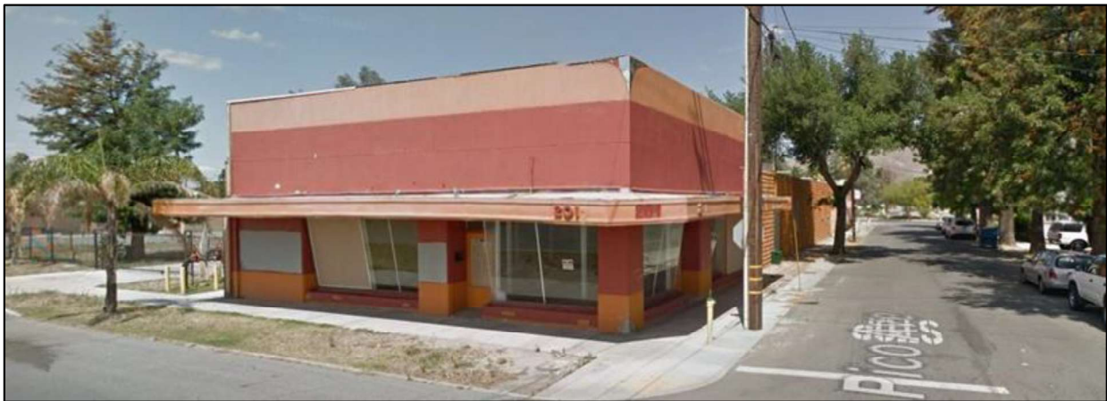
Mid-century Modern Commercial Building (1953) at 201 W. Main Street
