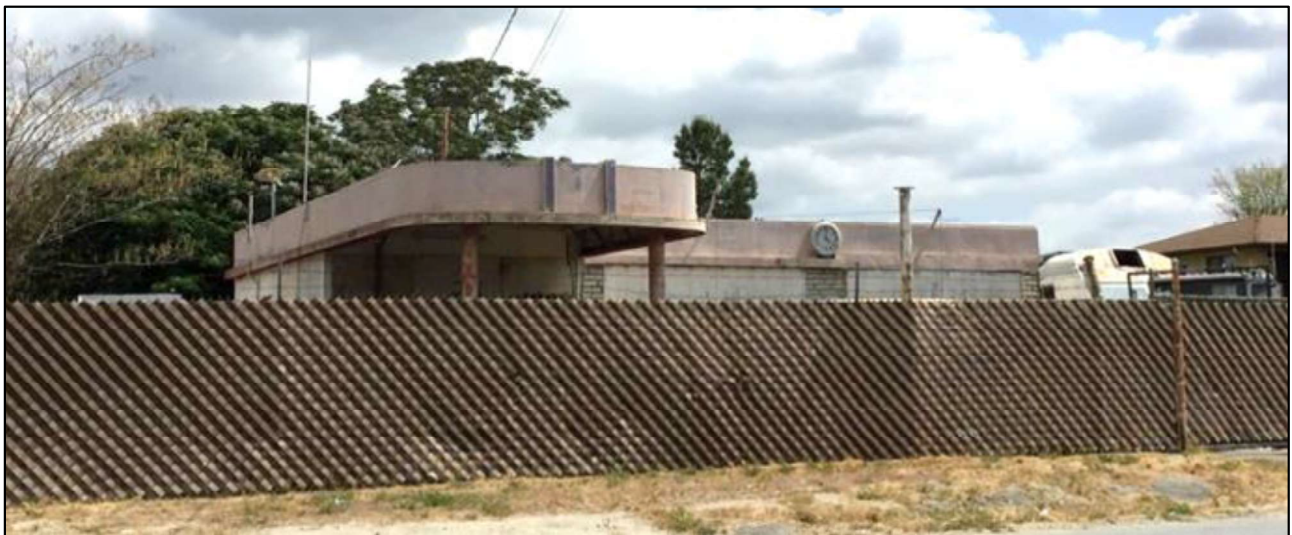
Figure 28. Streamline Moderne Gas Station (ca. 1930s) at 231 Idyllwild Drive
