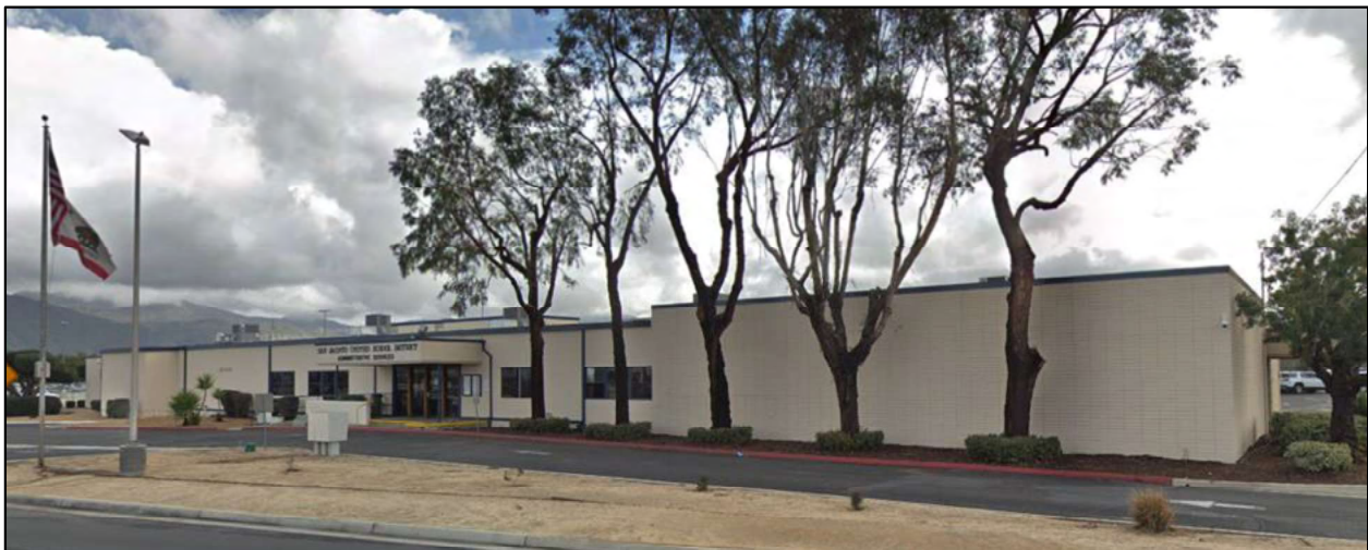
Figure 58. San Jacinto Unified School District Administrative Offices (1960s) 2045 S. San Jacinto Ave.
